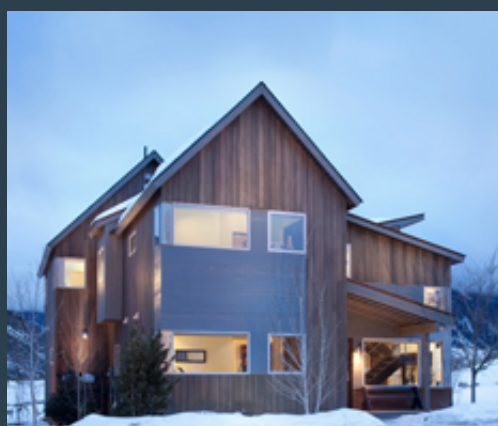
Burlingame Prefab – Aspen, Colorado
